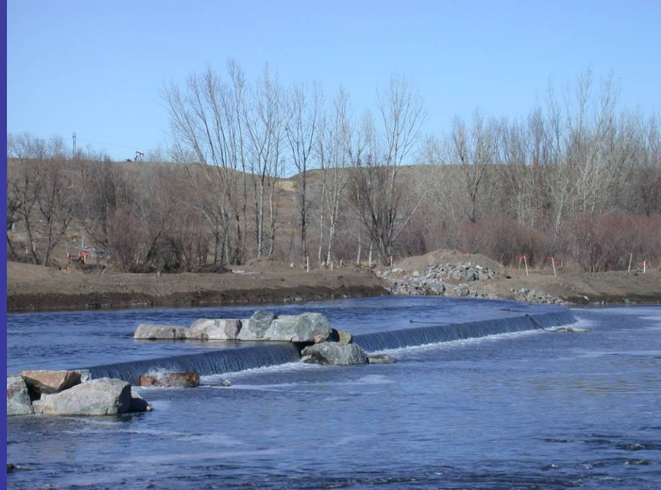
124 th Ave Drop Structure
